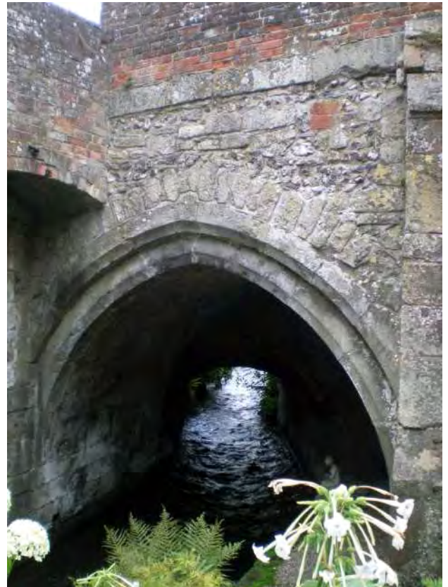
13th-century bridge under the B3046 in Alresford Photo © Pam Lang
